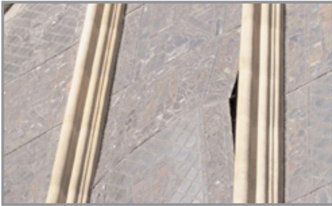
This article follows on (although belatedly) from the article about 'Replacing wire ties in situ' in issue 38 of June 2007, where Keith Hill addressed the difficulties experienced by glaziers/conservators when faced with the task of in-situ vertical soldering and replacing failed copper ties with new ones. Here we report another method of soldering wire ties in situ.
