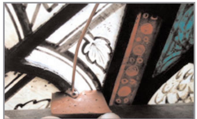
We soldered more additional ties than might normally be the case when, working on the bench, to help provide better long-term support. One mould stood up to being used about 40 times before it started to disintegrate. The rubber could also be held in place with the fingers if needed, as it is a good insulator against heat.
