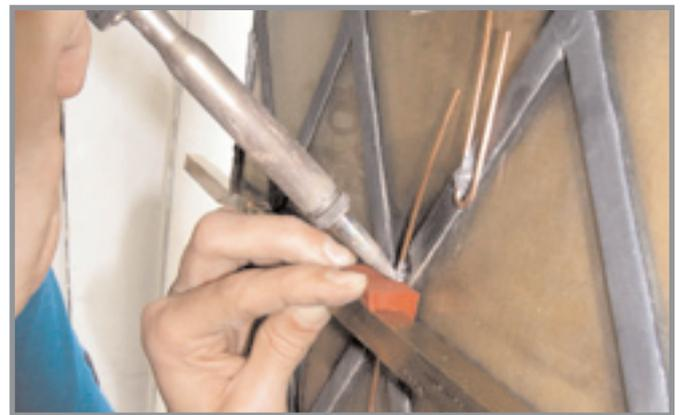
Though we found we could use a small micro-flame with caution, we favoured a 110 V – 100 W iron for the safety of the glass and the building. The mould allowed us to heat the solder for as long as it was needed for good solder-to-metal contact whilst holding the wire in place with pliers. The resulting solder blobs were reliably uniform and neat (photo below). We twisted the ties and folded them back on top of the bar so they were away from the risk of snagging and out of sight.
