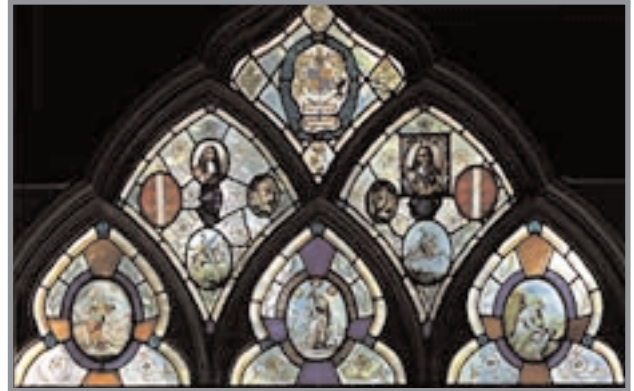
The Library window, July 2006, showing the 1950s layout of Miss Joan Howson, introducing out-of-scale borders in blue and orange around the three lower antique panels and a painted and stained background pattern of roses and foliage, which Dr Peover points out has no historical foundation. Moreover, the quality of glass painting is coarse and inexperienced, clashing with the refined, small-scale style of the antique originals from various centuries. After lengthy consultation with the architects and English Heritage, it was decided to discard the 20th-century backgrounds. ©Paul San Casciani
